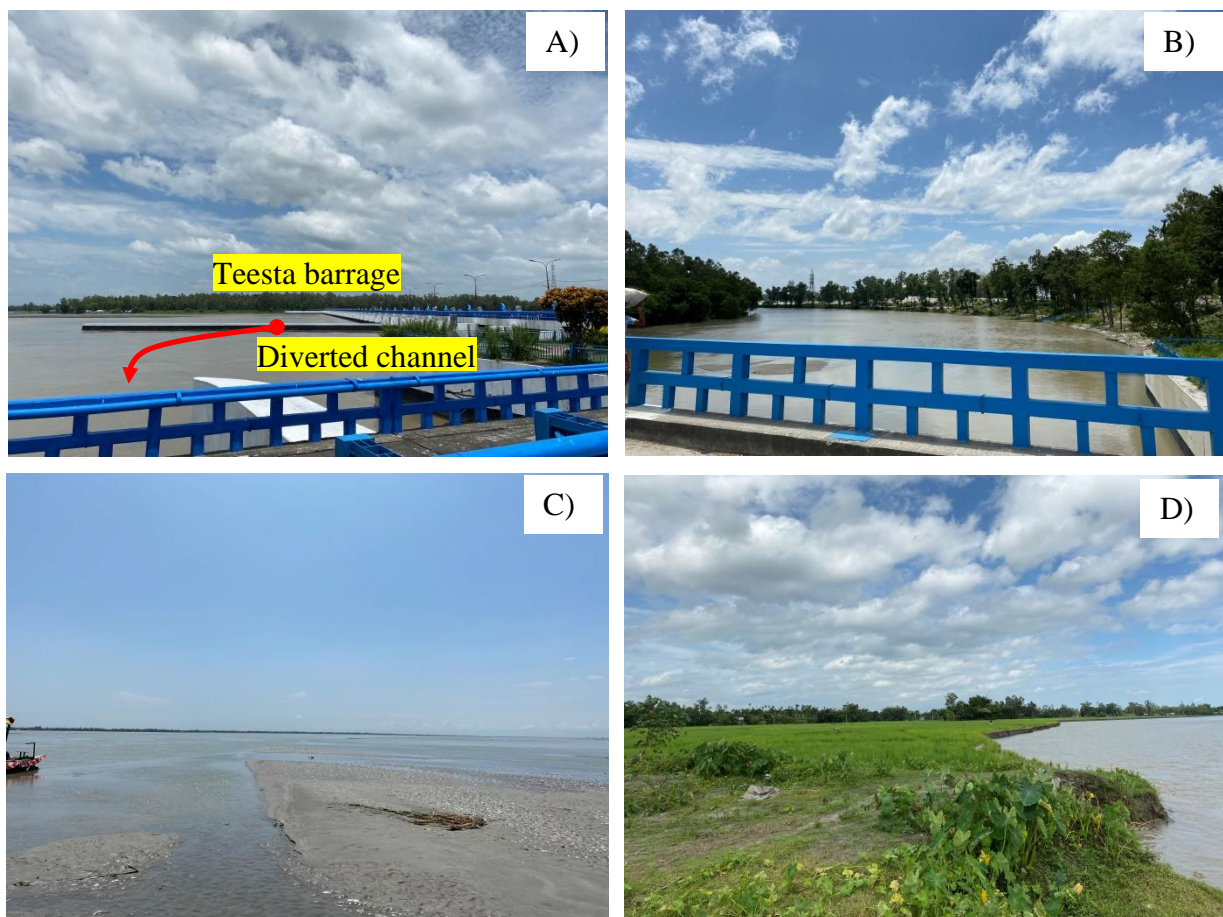
Fig. 3.15 A) Teesta barrage in Bangladesh, B) diversion of channel from the barrage for irrigation, C) deposition within the channel, and D) erosion along the bank.
