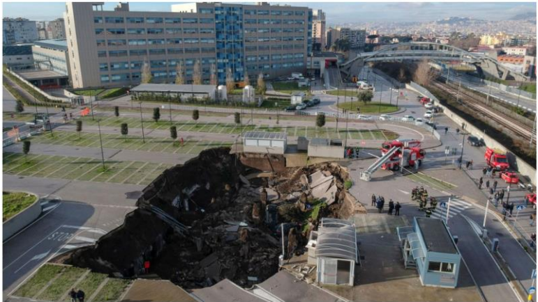
(b) Massive sinkhole near an Italian hospital in Napoli, Italy (2021). Source: CNN.
