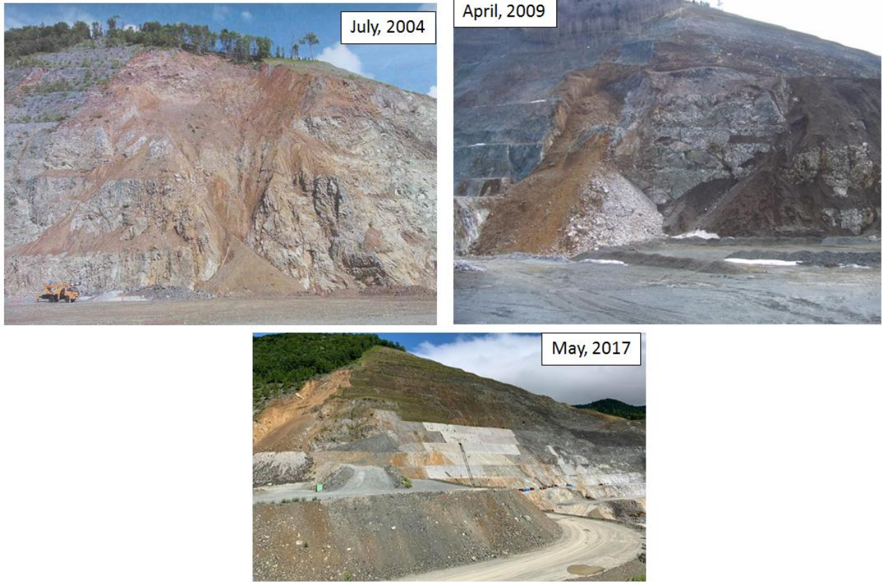
Fig.2.4: Plane view of rock slide that occurred at the quarry in 2004, 2009 and 2017.
