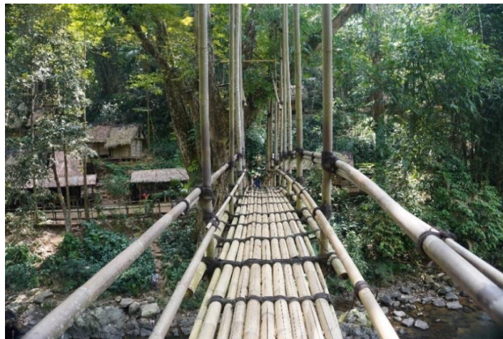
Figure 5.7. A Bamboo Bridge in Gajeboh Hamlet
