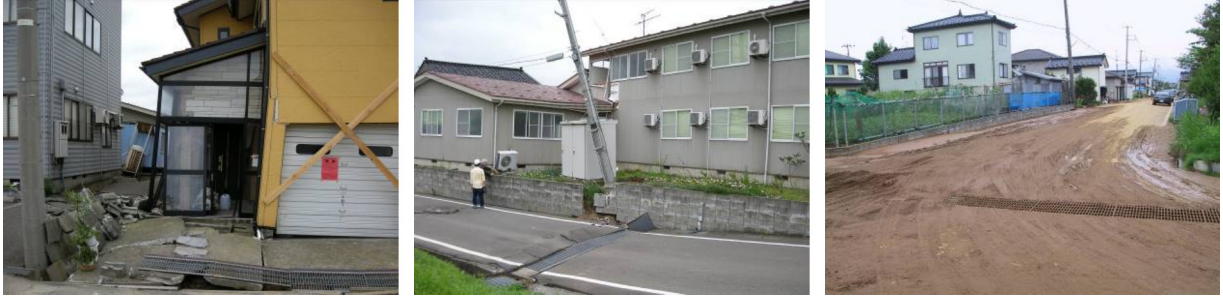
Fig. 3. Earthquake damage in Matsunami district of Kashiwazaki City: (a) most severely damaged house, (b) damaged houses due to ground crack, and (c) sand boiling (Isobe et al., 2014a).
