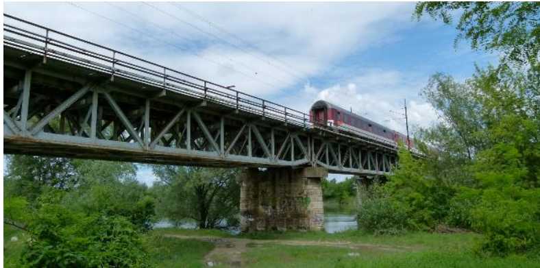
Figure 2. Side view of riveted truss bridge.
