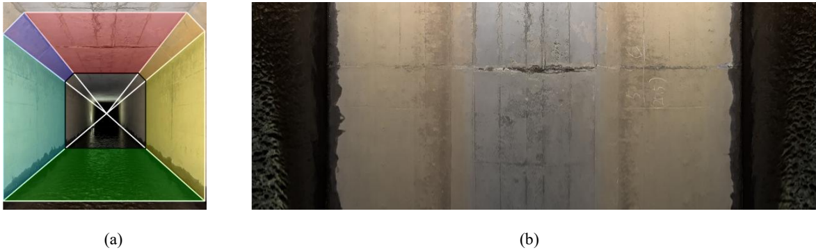
Figure 3. Wall face detection and unfolding result: (a) detected wall face regions with boundaries defined by the estimated vanishing point, (b) example of an unfolded wall face demonstrating that surface detail is preserved after perspective correction.
