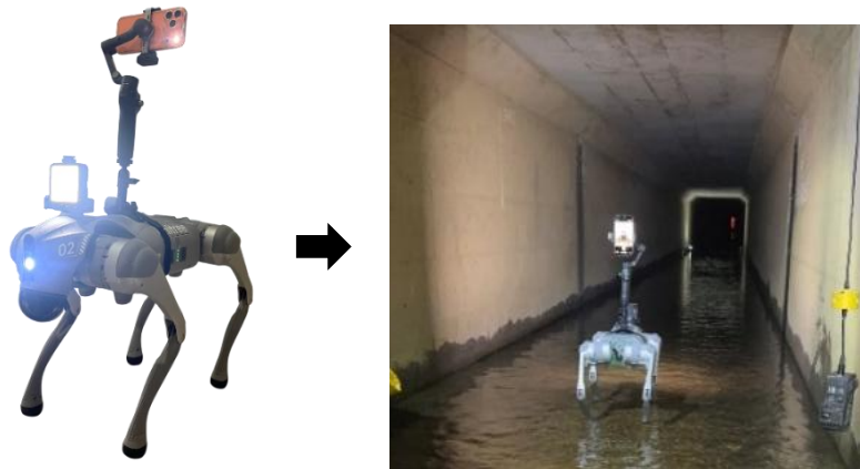
Figure 1. The quadruped robot deployed inside the underground box culvert during field inspection, showing the inspection environment, water accumulation, and camera-lighting configuration mounted on the robot.
