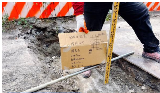
Figure 5. Photograph showing the box culvert identified in Area A.
