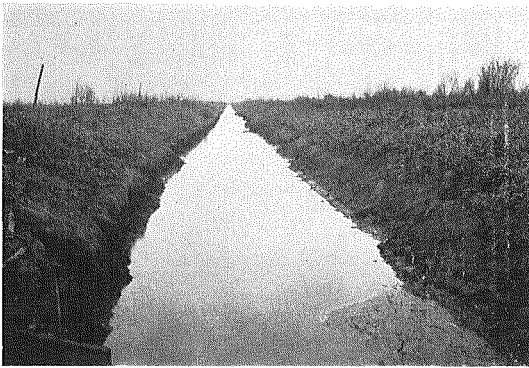
Photo. 3・1. Excavated channel before lining
