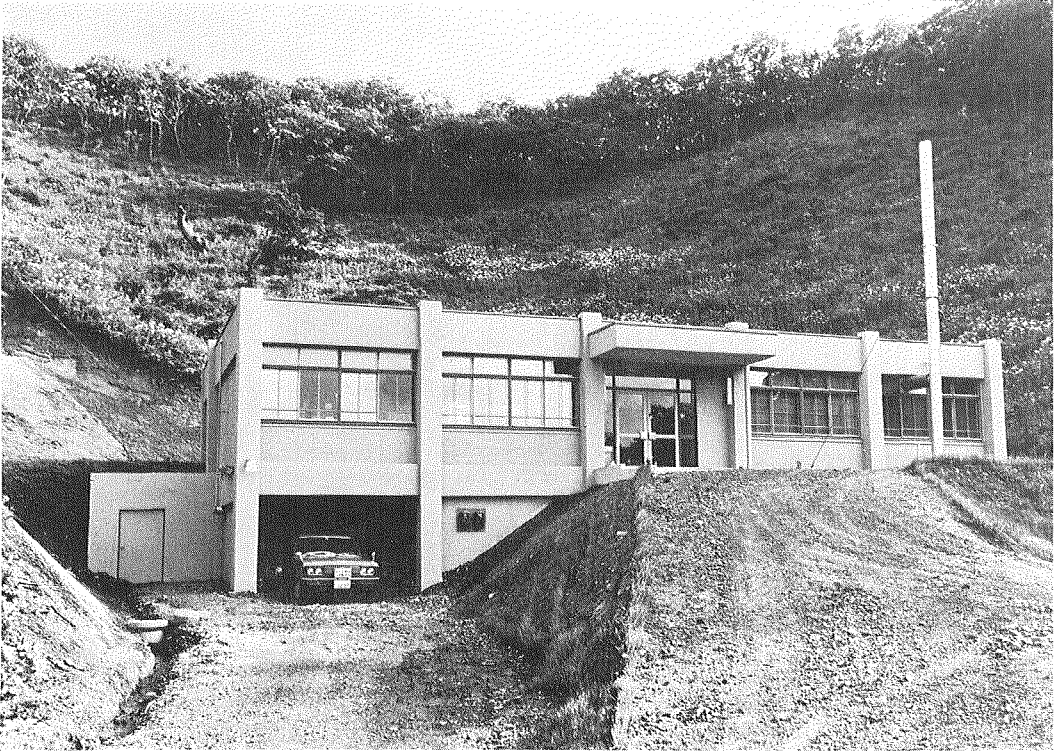
Photo. I. An outside view of the Erimo Geophysical Observatory. On the left side of the observatory there is the entrance of the observation gallery.
