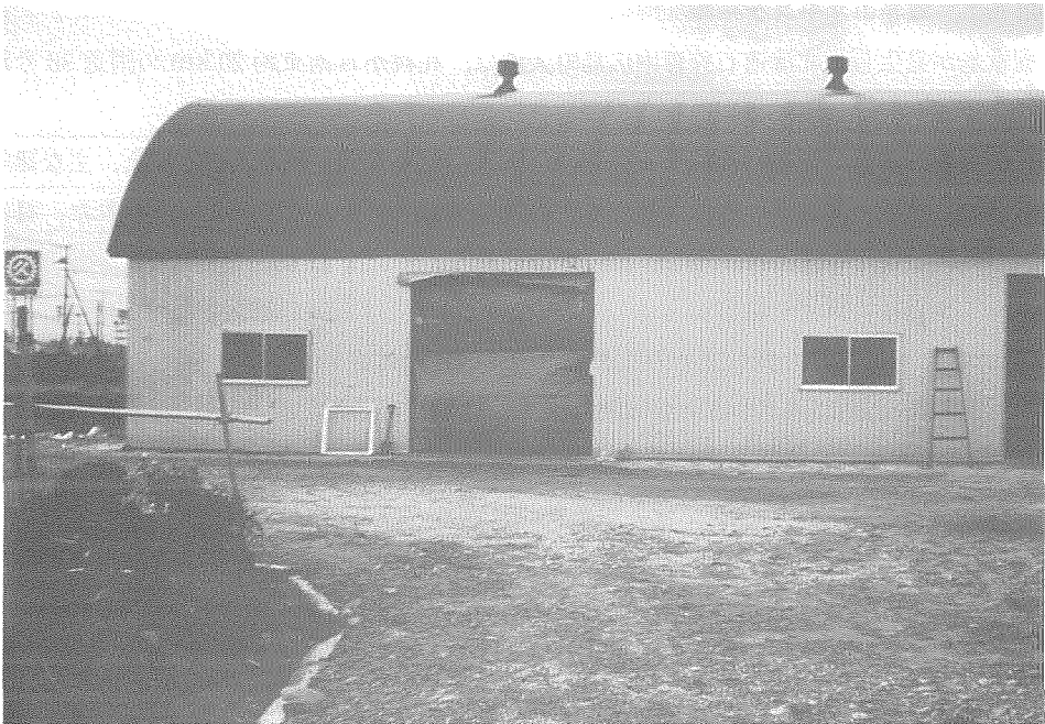
Fig. 2. A warehouse which two shutters were taken off and blown away.
