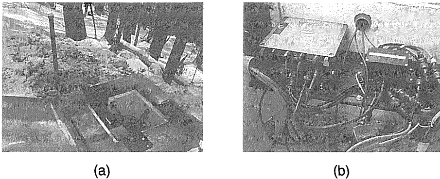
Fig. 3. (a) Overview of the MTU-5 unit installed in concrete bunker at Esashi observatory. Recorded magnetic and electric time series data at both observatories are synchronized by GPS clock (central part). (b) Observed data are recorded to the MTU-5 box (left side) and transferred to the external PC every hour through the Fax modem (right side).
