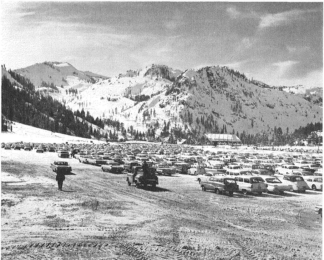
Fig. 1. Compacted-snow parking lot protected with sawdust at Squaw Valley, California
