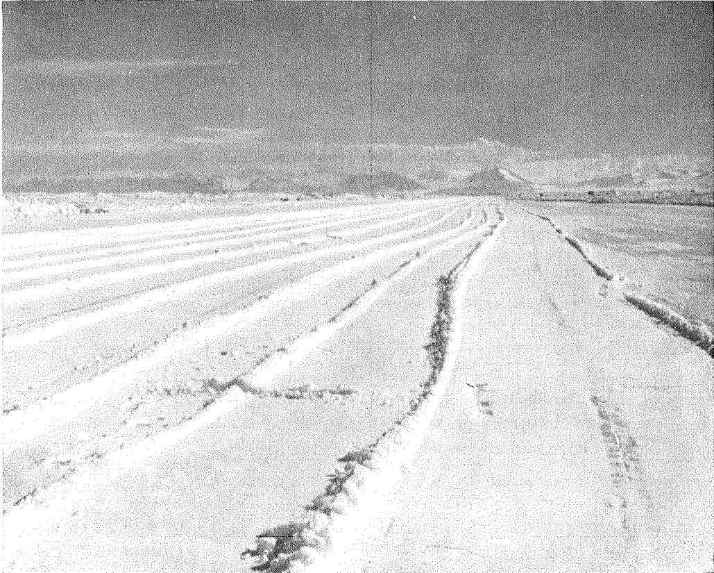
Fig. 7. Pulvixed ice surface on left and untouched ice on far right at McMurdo Station, Antarctica sea ice runway
