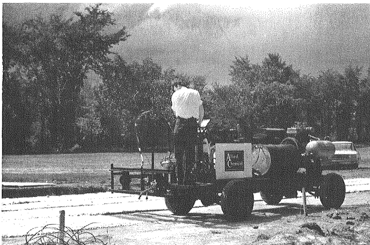
Fig. 8. Self-propelled foaming machine in operation
