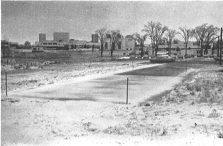
Fig. 12. Snow remains on insulated surface as evidence that after a cold period, surface temperatures on insulated area are colder than on non-insulated area
