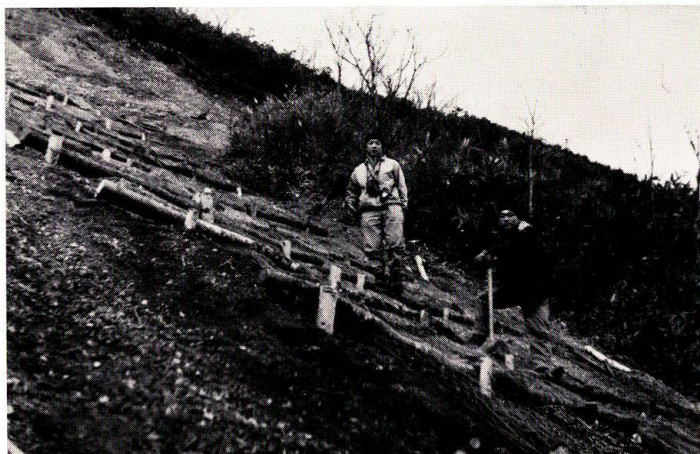
Plate 2-2. Spread nettings are settled by means of poles on the slope.
