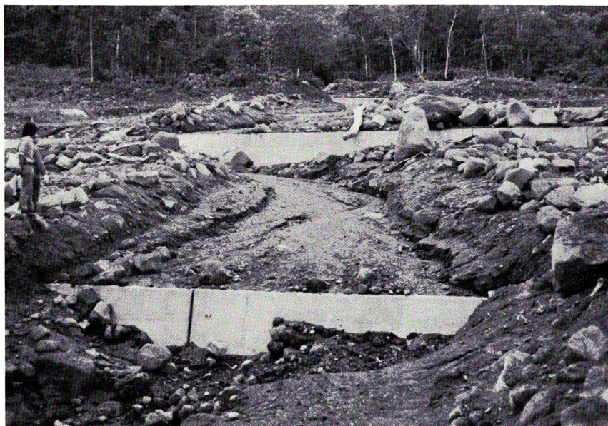
写真—5 床固工群による土石の分散堆積 (青木の沢扇状地, 1975, A 堆積地) Photo 5. Despersion of Debris Flow by the Groupe of Soilraining Works (Aokinosawa Fan, 1975, A-deposit).
