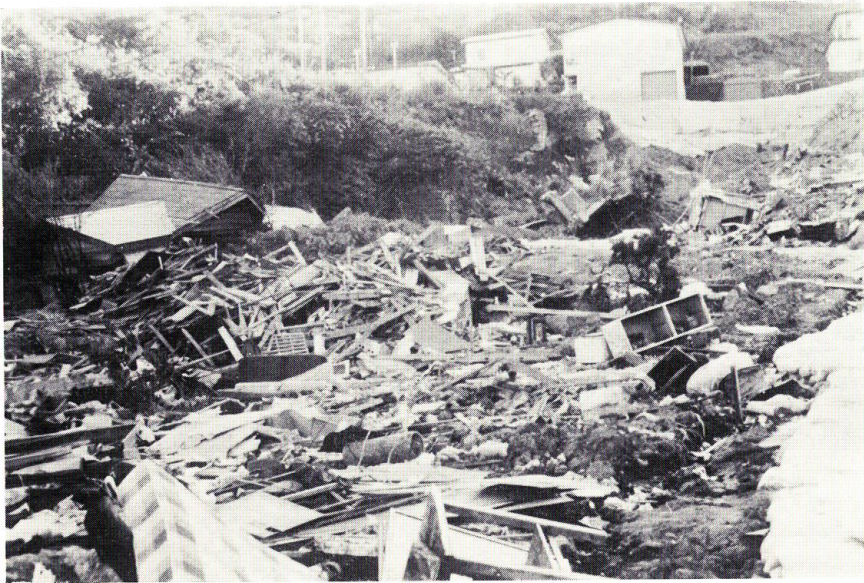
Photo 1. Failure of housing site prepared by filling up vally in Ōsawa-chō, Muroran city. The filled earth broke down as debris flow razing 6 houses and burying 3 houses and the original stream bed appeared.
