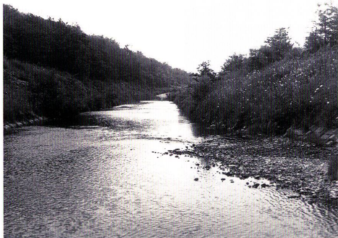
写真三 改修区間の溪相(積丹川) Photo 3. View of the altered section in the Shakotan river.
