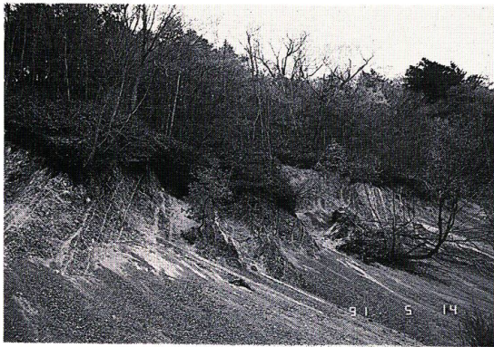
Photo 4. View of Streambank Collapse in Upstream Part of Atsuma River Basin
