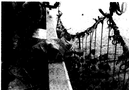
Fig. 70. Condition of the air bag attachment on the main line.
