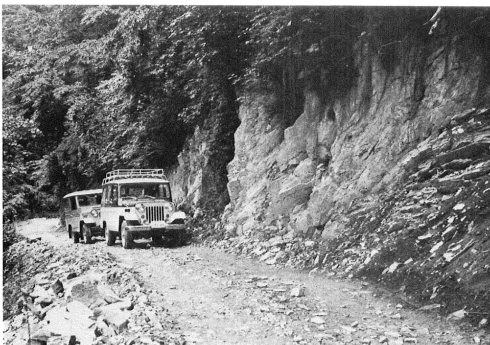
Plate 1 Surveying in the road between Tyoanji and Ohno. The instrument is mounted on the front jeep.
