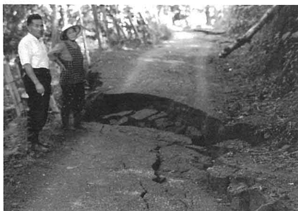
Text-fig. 6 A normal fault cutting a trail in the atrio, observed at 0850, 20 min. before the beginning of eruption on August 7, 1977. (photo by courtesy of Mr. Ishibashi)
