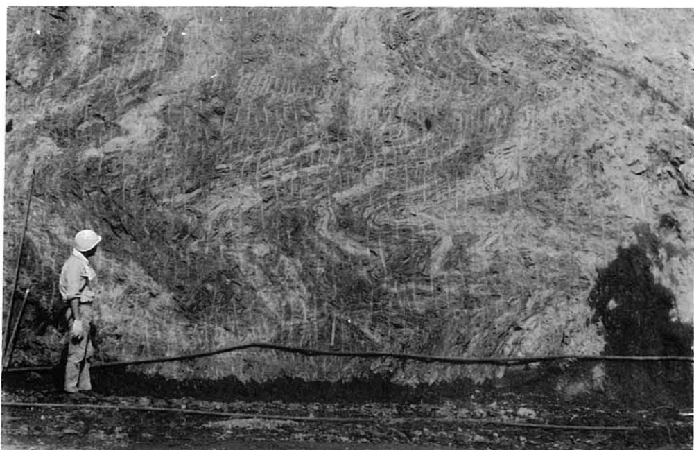
Text-fig. 9 Photograph of "Shear zone-A" at the northern side of the Iwaonai damsite. The folded strata are regarded as Cretaceous turbidite cataclasite from the lithological feature. Microfolding axes run N70^{\circ}E . This photograph was taken in 1966 during the construction of the dam. On the right side, out of sight, "Zone of breccia" appears.
