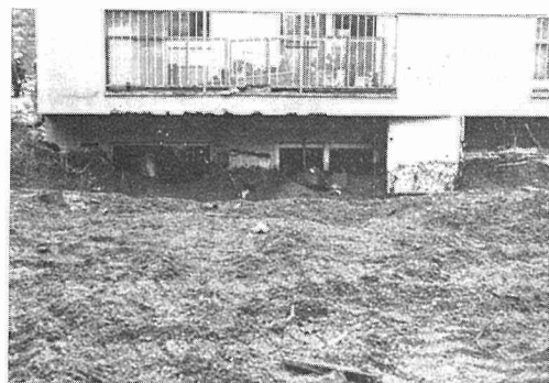
Photo 8. The ground floor of a three-storied apartment house, which is seen in the rearmost right in Photo 7, was penetrated and completely buried by the mudflow of new tephra with a depth of more than 2.5 m.
