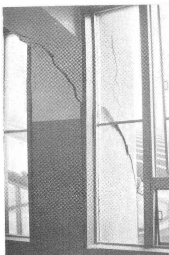
Fig. 14. Second story column in North-west Wing
