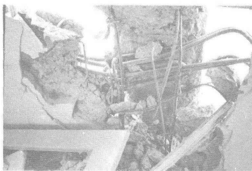
Fig. 10. Wall-girder — pilaster joint
