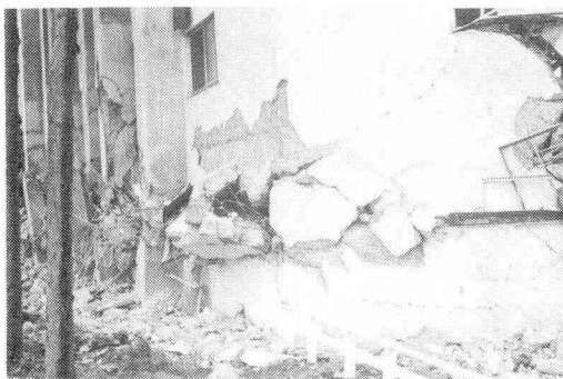
Fig. 16. External wall in the bend
