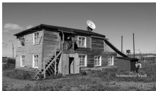
Photo-11. Station OHT is located at Okhotsk Aerological Observatory. The seismometer vault is adjacent to the observatory.
