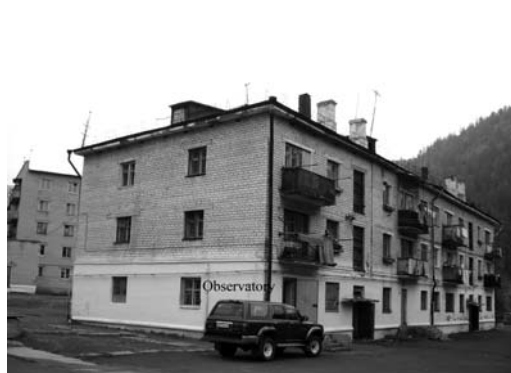
Photo-7. Station GOR is located at Gorney Seismic Observatory belonging to Sakhalin Experimental Methodical Seismological Department. The seismometer vault is in the basement of the observatory.
