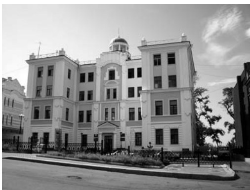
Photo-6. Station KHA is located in a building of Institute of Geography in Khabarovsk. The seismometer vault is of the basement in the building.
