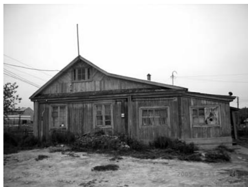
Photo-5. Station OKH is located at Okha Seismic Observatory belonging to Sakhalin Experimental Methodical Seismological Department. The seismometer vault is in the basement of the observatory.
