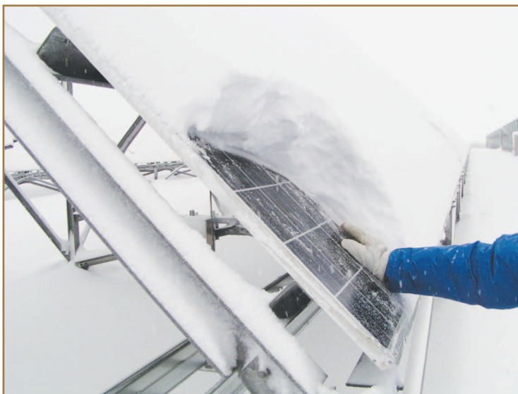
figure 14. Snow accumulation on the PV array.
