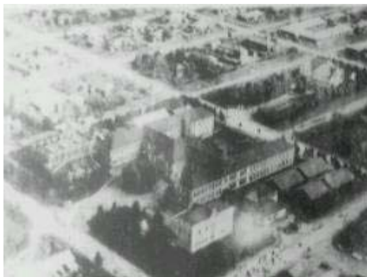
Fig. 5. The Karafuto-Cho Office Building (a. 1908)
