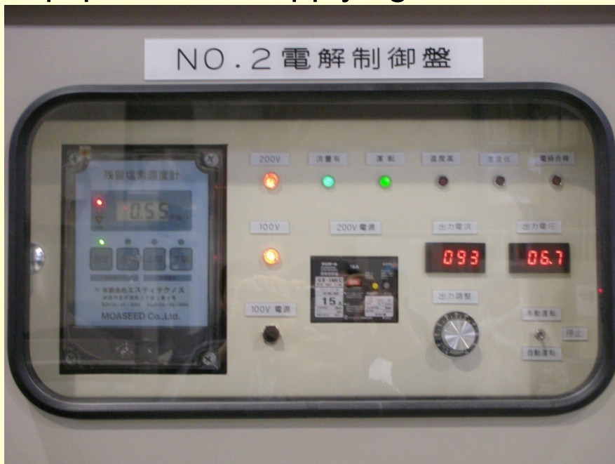
Equipment for supplying a disinfected seawater, (disinfection rate 0.55 mg/L, 99.8 %)
