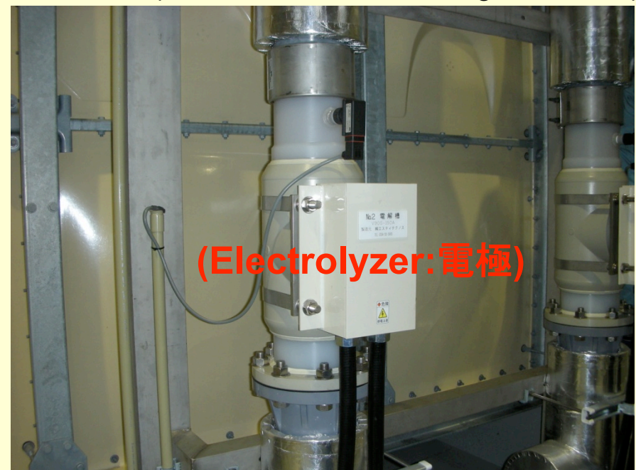
Equipment for supplying a disinfected seawater, (disinfection rate 0.55 mg/L, 99.8 %)
