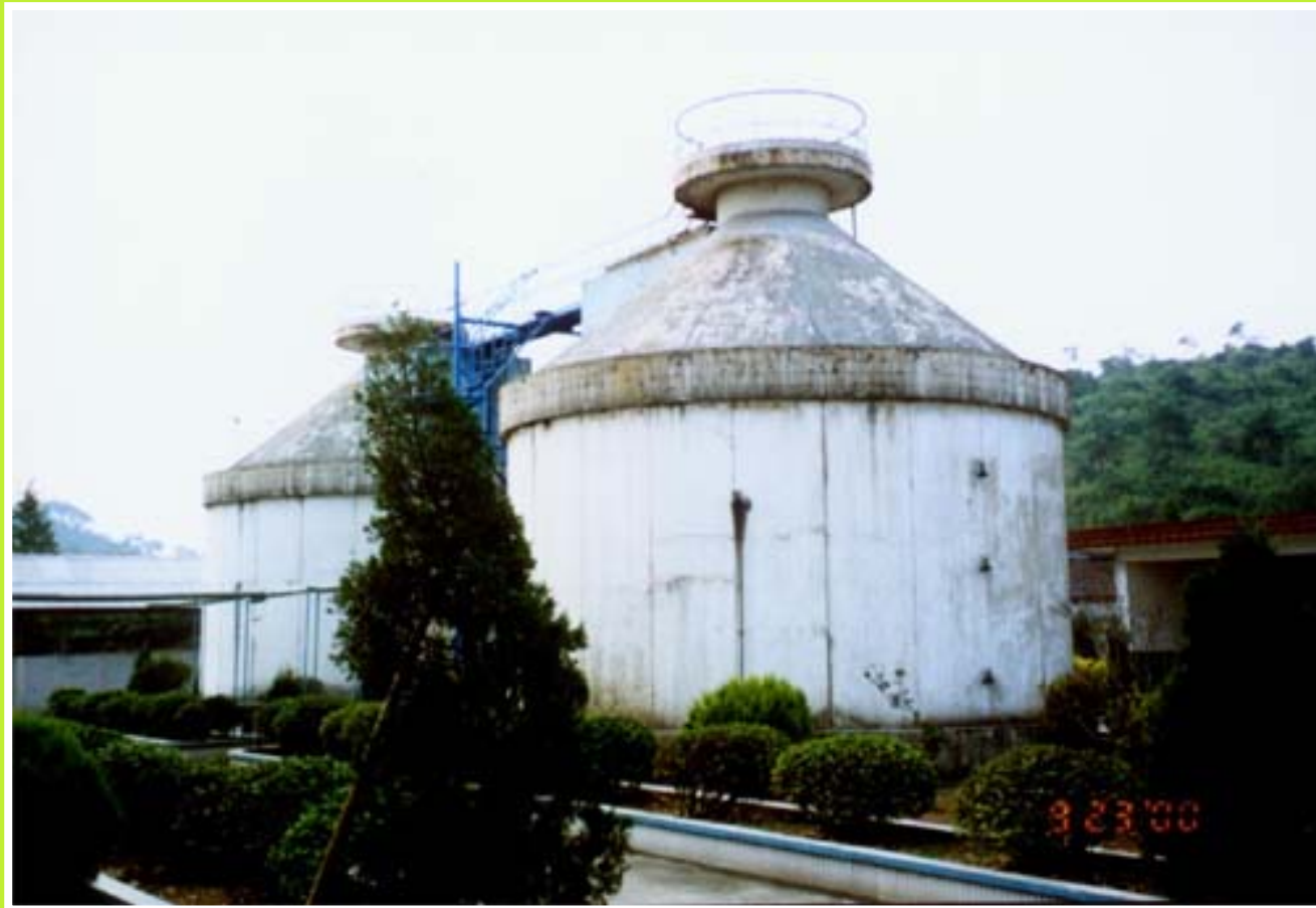
The biogas digesters in Fushan Integrated Ecological Farm
