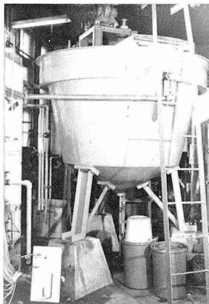
Photo 1. 30 m 3 /day floc blanket type suspended solids contact clarifier.
