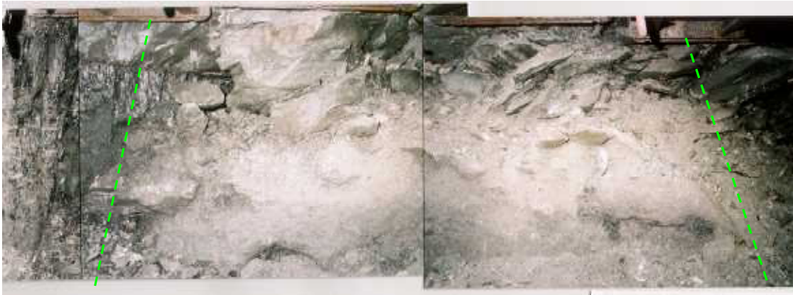
Fig. 9 Old roadway observed in Jobu Hidari No. 5 SD. Old roadway was closed by the deflected and sagged roof. Rocks below the deflected roof were softened.
