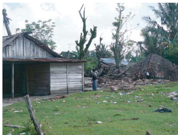
Fig. 1. Photograph of a house near the Tiku XDR site that was destroyed by intense wind on November 19, 2006.
