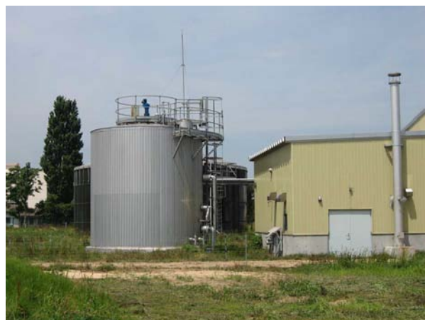
Fig. 4-31. Biogas system with methane fermentation.
