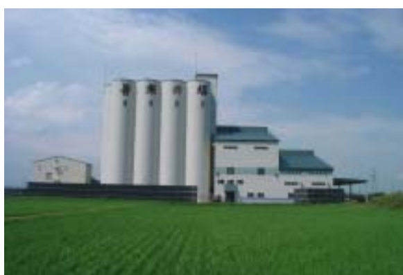
Figure 2. Side view of Uryuu grain elevator. (The silo on the left is one of the silos used in the experiment.)
