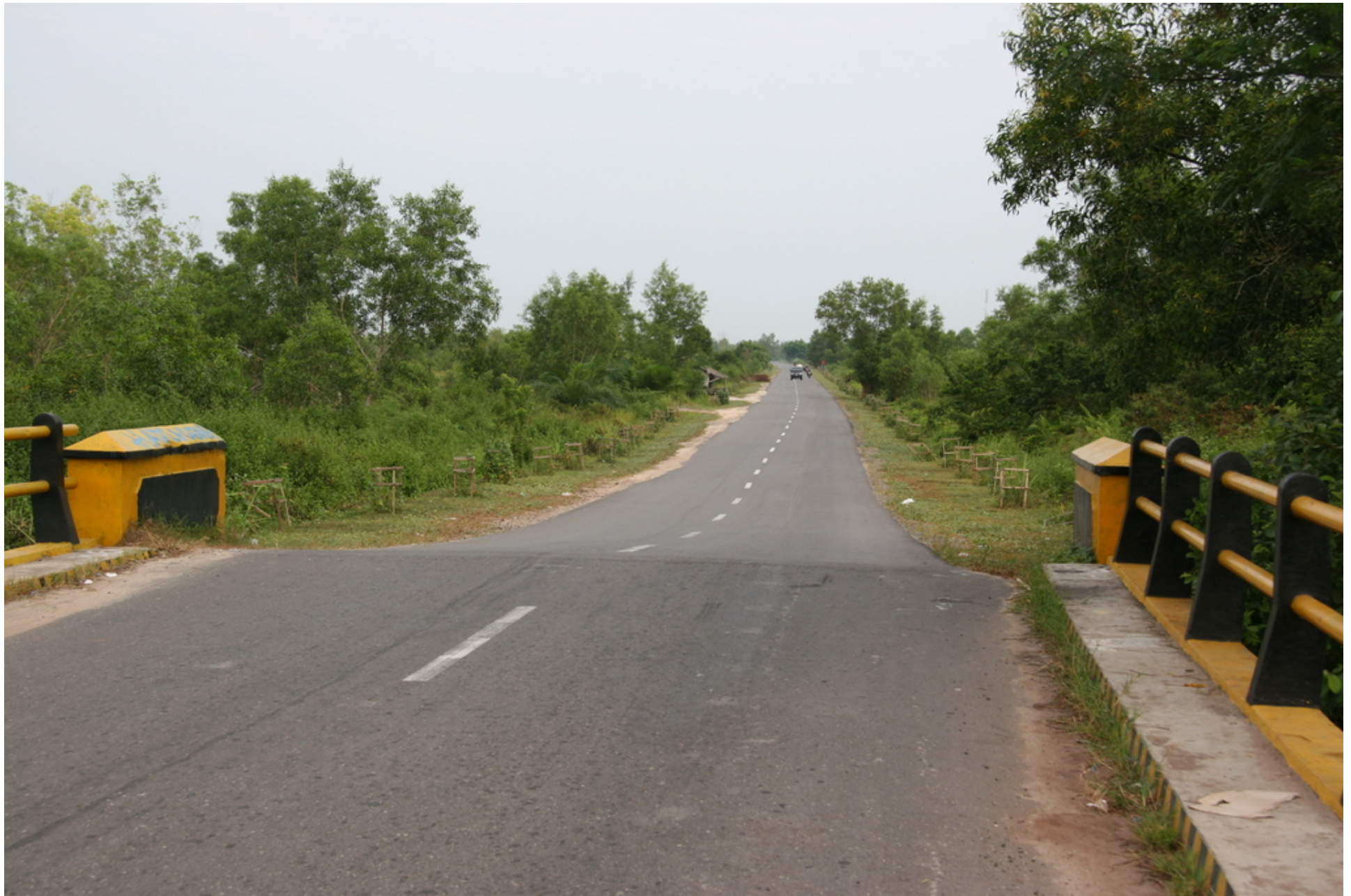
Canal Bridge, Kalampangan, Central Kalimantan
