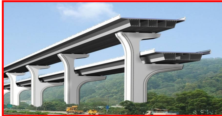
Figure 1 the F-bent double decked bridge column
