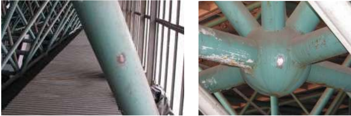
Figure 4: Preparation of surface of measuring bases on verified members.
