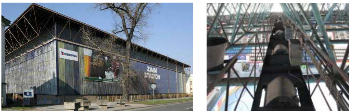
Figure 2: Winter sport stadium in Olomouc city – overall view and roof structural system.
