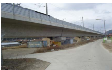
(a) Imgi 2 nd Bridge
