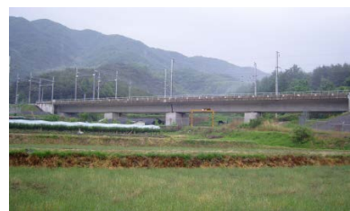
(b) Maeaji Bridge
