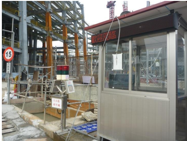
Figure 2: Installed RFID devices in the construction site.
