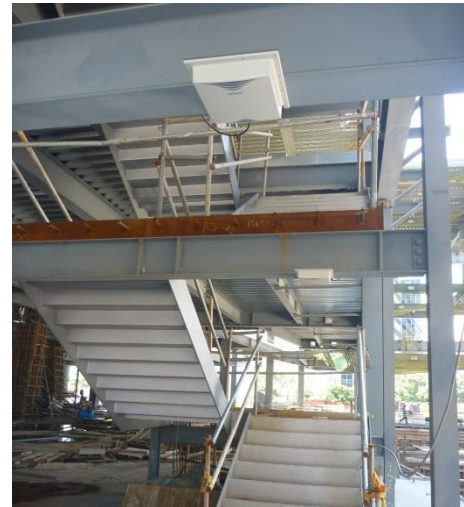
Figure 2: Installed RFID devices in the construction site.
