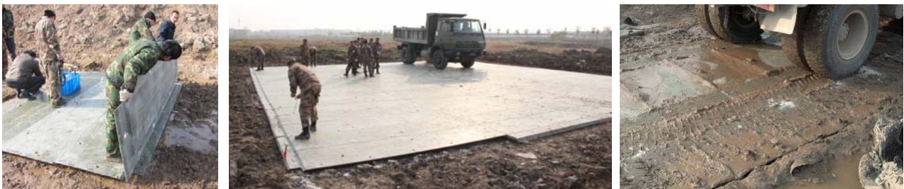
Figure 4: Composite pavement matting.
