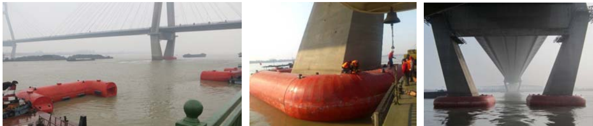
Figure 9: The North Bridge of Runyang Bridge composite collision avoidance facilities.
