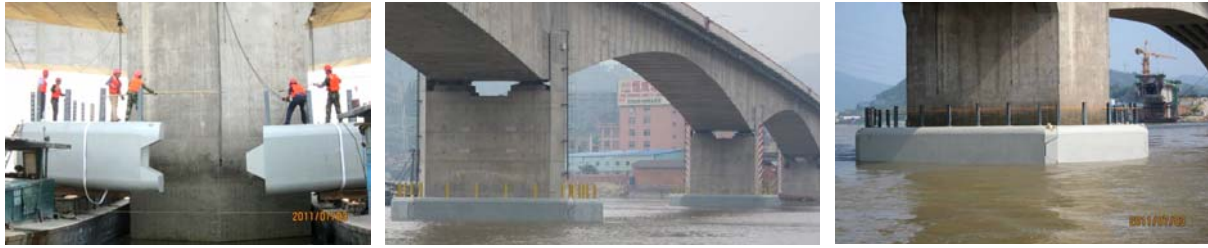
Figure 8: Fuzhou Wulong River Bridge composite collision avoidance facilities.
