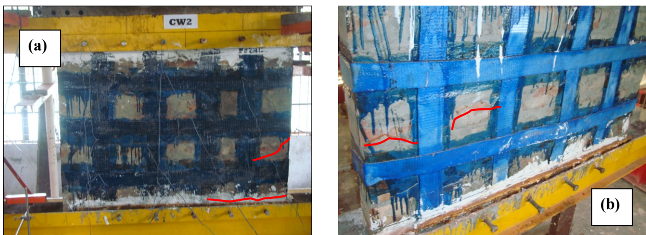
Figure 9: a) Failure at wall CW2 and b) PW2
