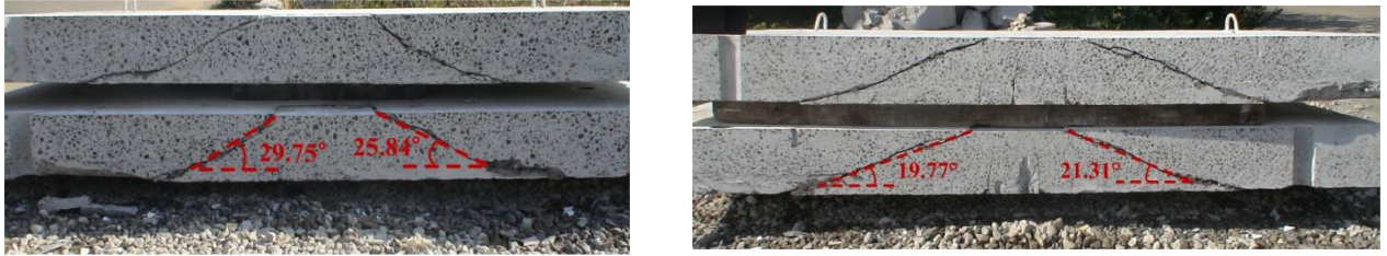
Figure 4 Punching shear failure surface: (a) LA Specimen; and (b) LD specimen.
