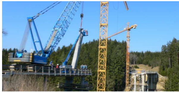
Figure 5: Vertical assembling of the arch
