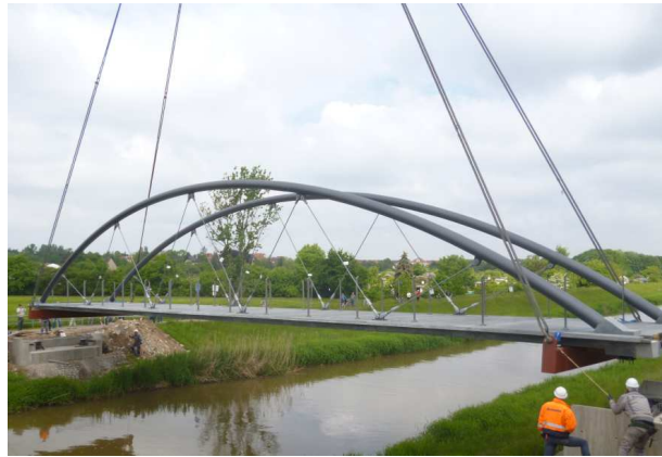
Figure 11: Assembly of the bridge with mobile crane
