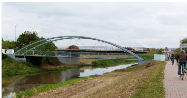
Figure 9: Hybrid footbridge Markkleeberg
