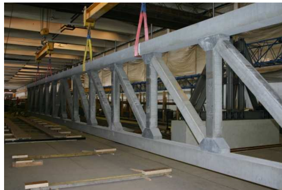
Figure 7: Truss construction for the full scale test
