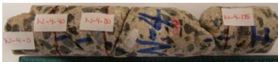
Figure 1: Core sample from RC column after fire test.
