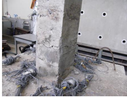
Figure 7: Cracks at plastic hinge zone
