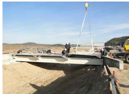
Figure 9: Erection of deck panels.
