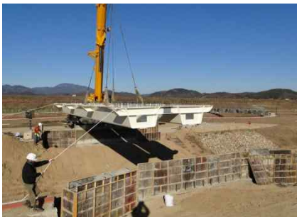
Figure 8: Erection of U-girder.
