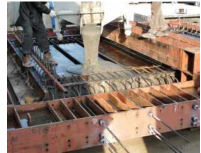
Figure 7: Placing of UHPC.
