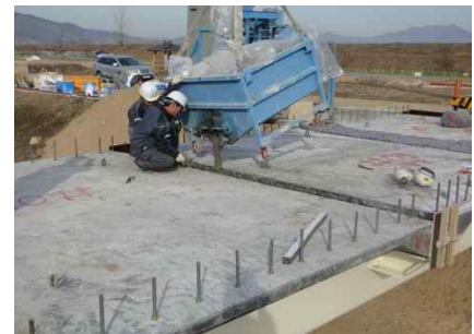
Figure 10: Placing of UHPC joints.
