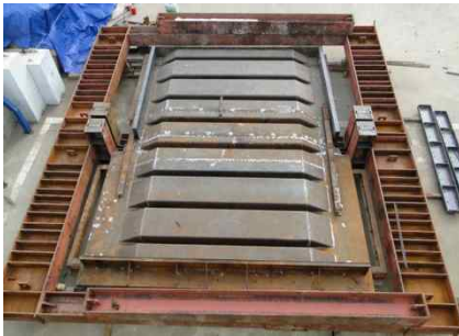
Figure 5: Assembling of prestressing table and deck form.
