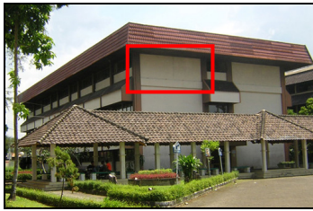
(a) RC building with brick masonry infill
