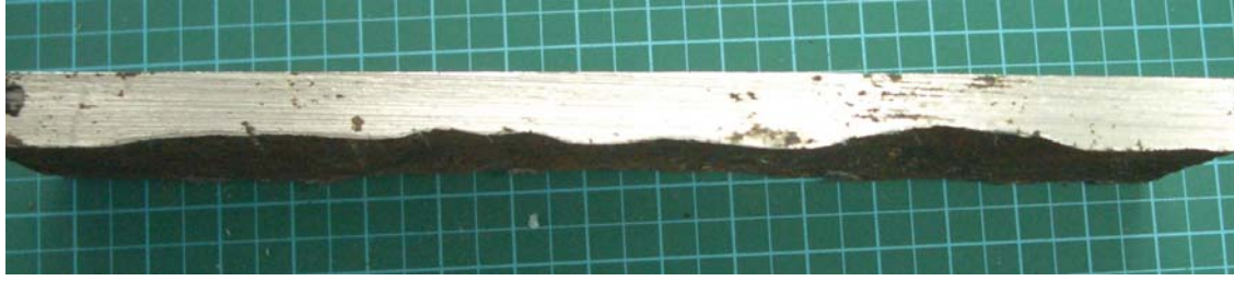
Figure 8: Corrosion inspection specimen from Benoki Bridge (Okinawa) web plate.
