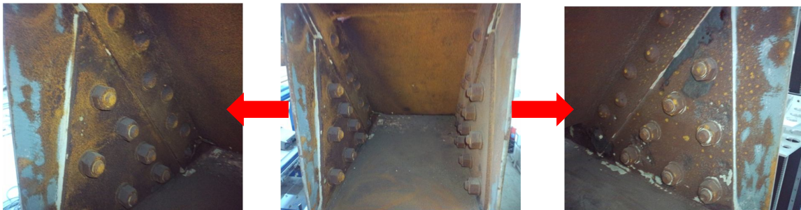
Photo 7: Inner surfaces of P72u connection
